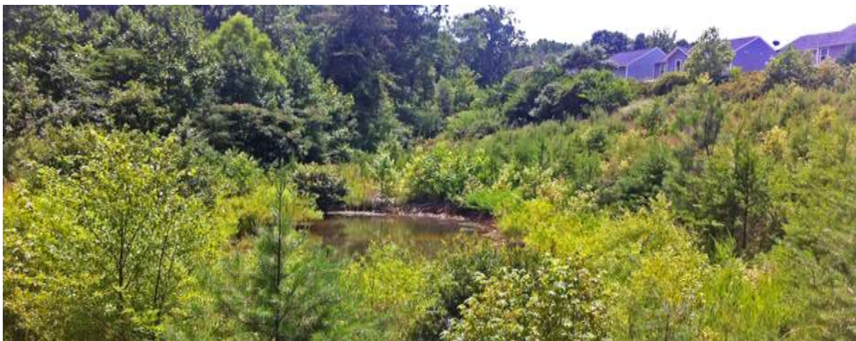
This neglected stormwater pond elsewhere is overgrown with vegetation and has lost its hydraulic function.
