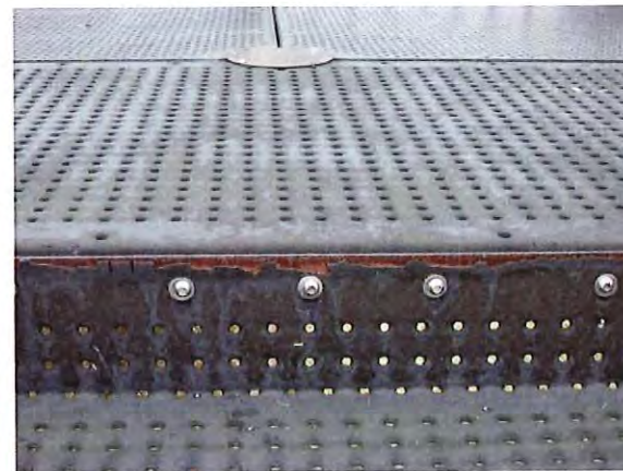
Rust and finish deterioration at steps
