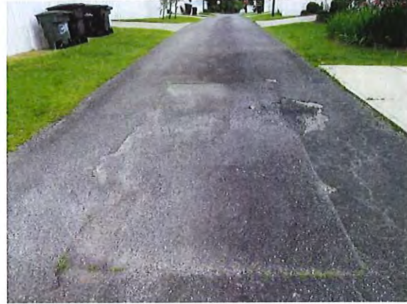
Pavement cracks and deterioration
