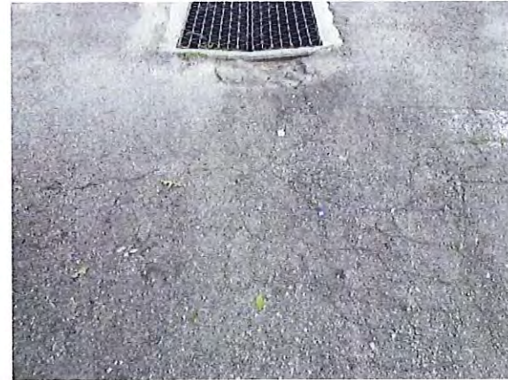
Pavement cracks
