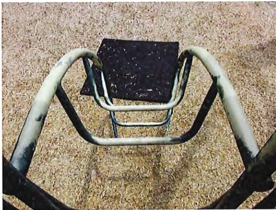
Stairs at main equipment – finish deterioration
