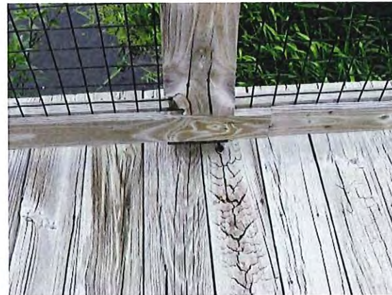
Bridge 2 deck board deterioration
