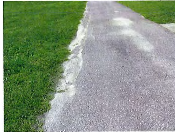
Asphalt walking path edge deterioration near playground
