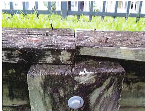
Displaced top board with exposed nails
