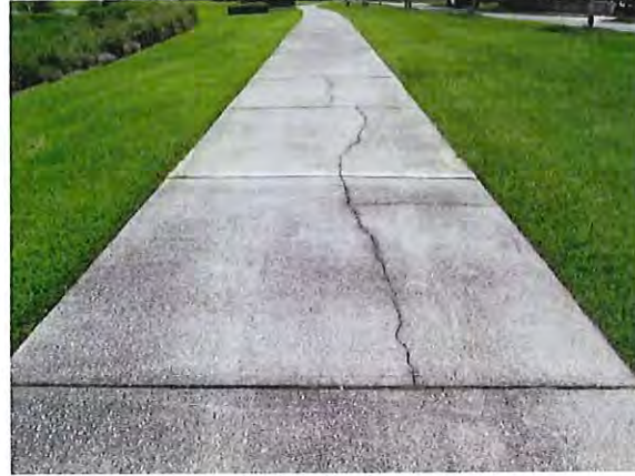
Crack at concrete walking path
