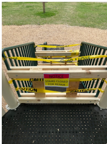
Figure 3 Main staircase after barricade
