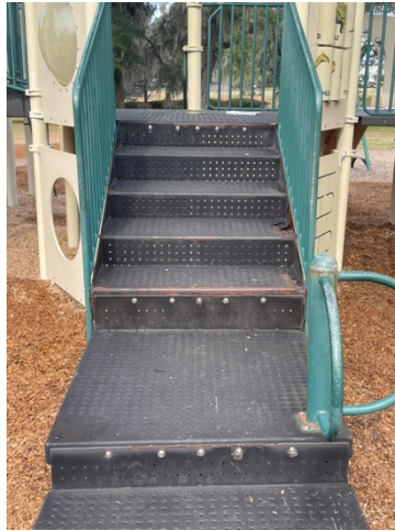
Figure 1 Main staircase before barricade
