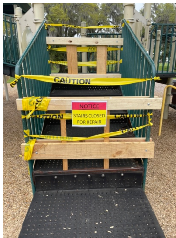
Figure 2 Main staircase after barricade
