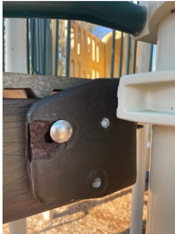
Figure 5 Existing bridge bracket
